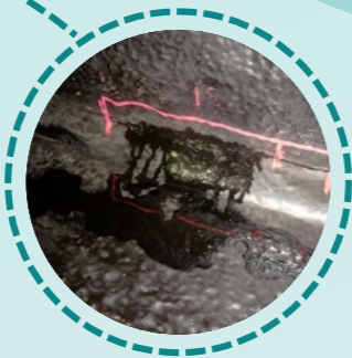
Example of a crude oil leak repaired on a FPSO in South-East Asia
