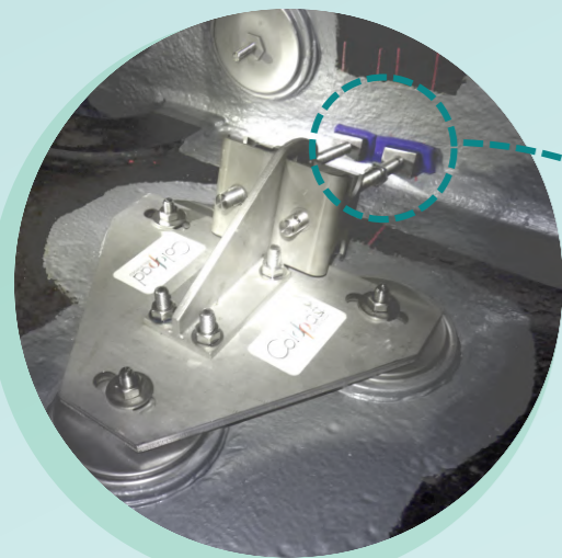
Example of a crude oil leak repaired on a FPSO in South-East Asia
