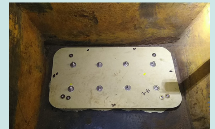
New plate bolting and filler pouring
