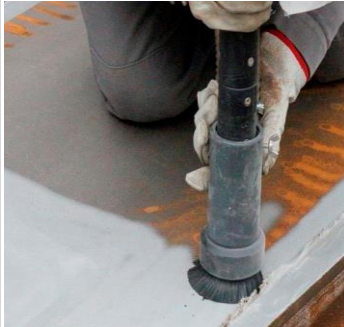
4- Then, the two-step Offshore Installation Process is carried out: A qualified Surface Preparation is performed prior to the Vacuum-Assisted Injection of the structural polymer (epoxy resin).
