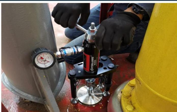
Proof load testing
