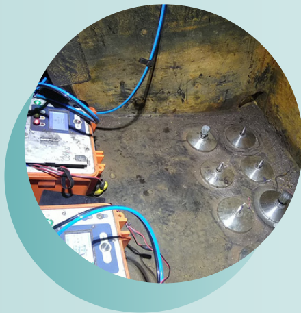
Bonding of C-Claws on the corroded area.
