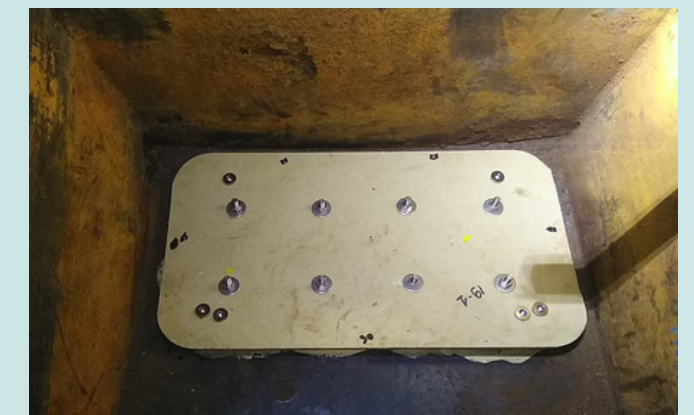
New plate bolting and filler pouring
