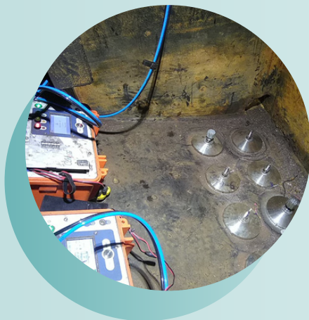
Bonding of C-Claws on the corroded area.
