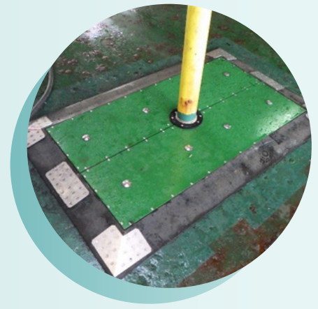
Steel plate to protect the area from further corrosion.
